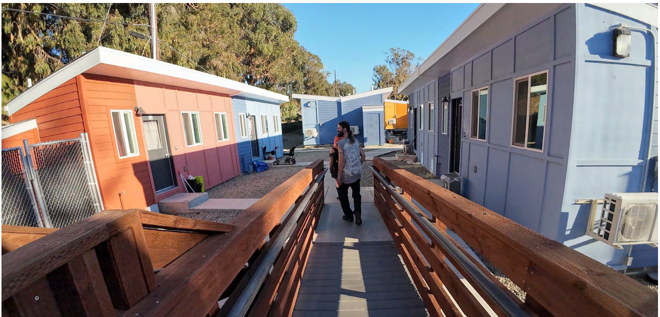
Fairmont Navigation Center, San Leandro
