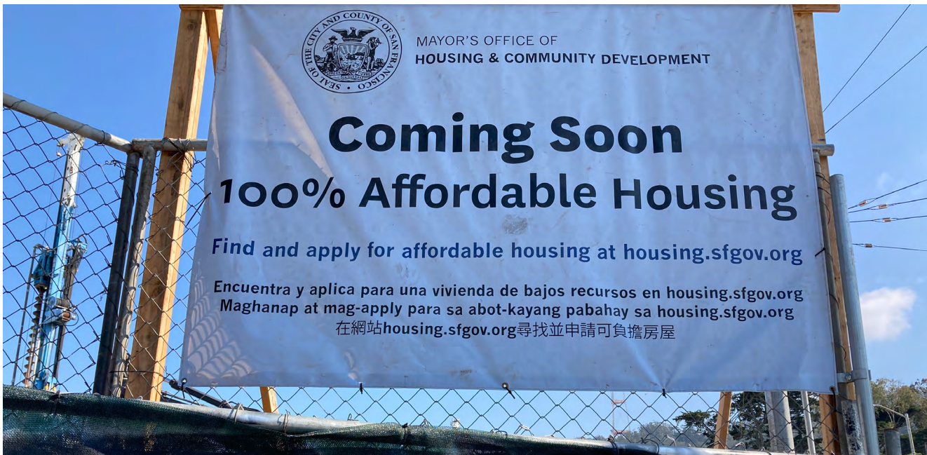
Affordable housing construction site, San Francisco Photo: Joey Kotfica
