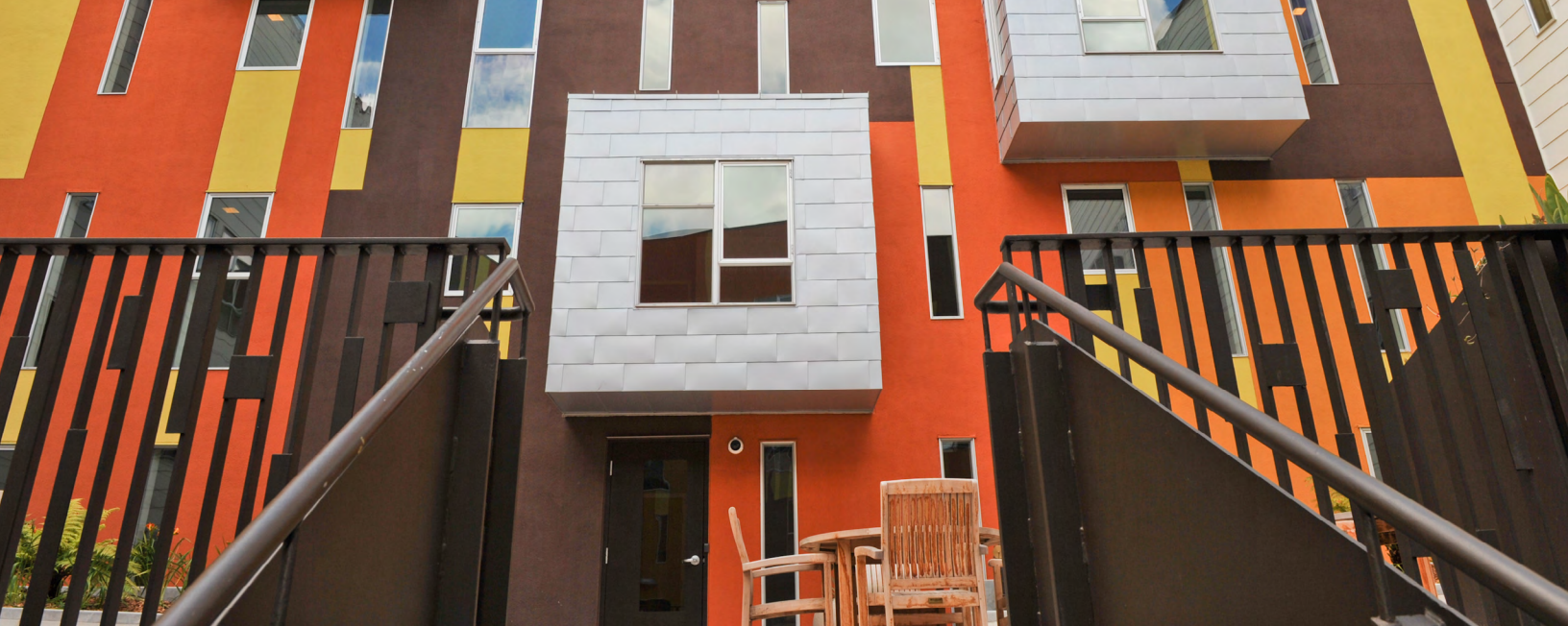
Armstrong Place Senior Housing in San Francisco Photo by Julio Cesar Martinez, courtesy of BRIDGE Housing
