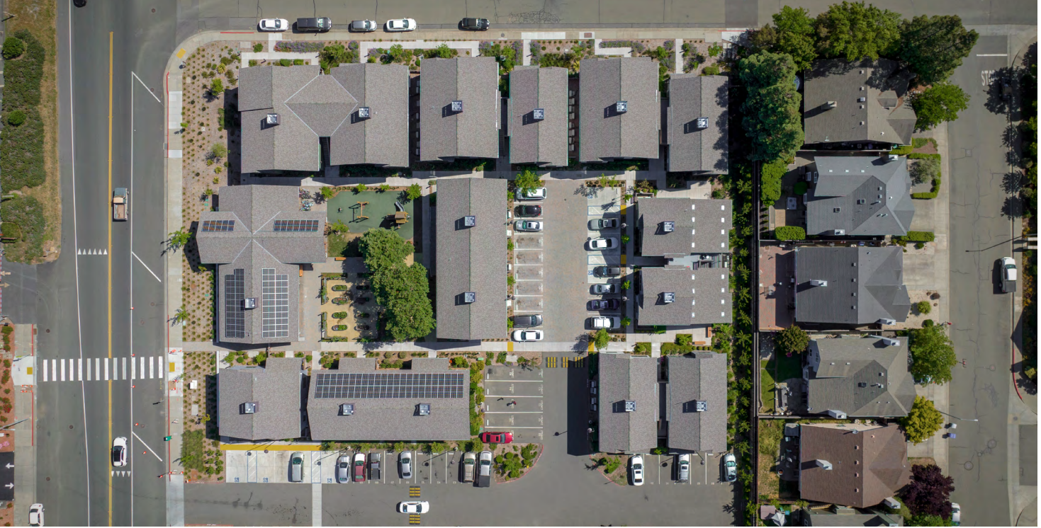
Residential housing, Sonoma County Photo: Karl Nielsen
