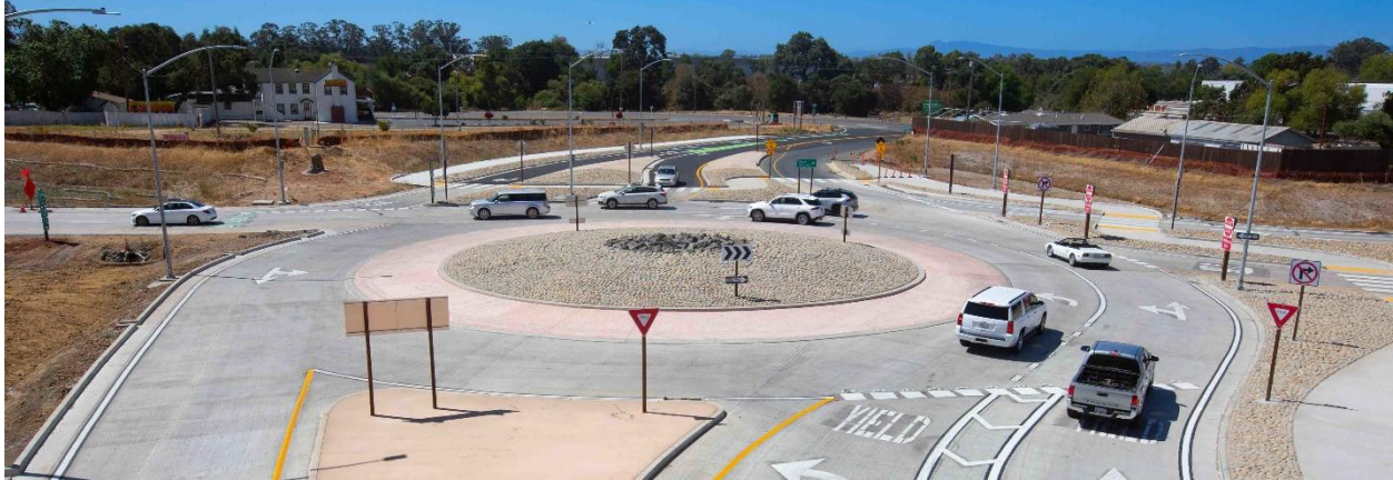
SR 29/Soscol Junction. Top: Photo of Soscol Junction Roundabout. Left: Photo of Soscol Junction Flyover Connector. Right: Photo of Soscol Junction bike lanes. Photos: Napa Valley Transportation Authority
