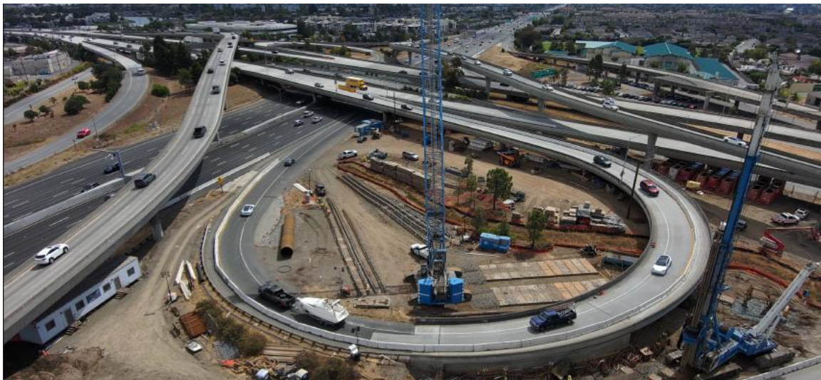
US 101/SR 92 Construction Progress SMCTA Photo
