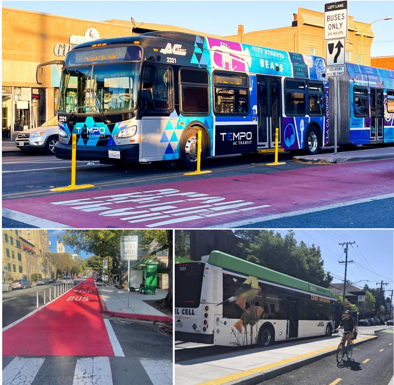
Quick Build improvements and bus delineation on International Boulevard in Oakland (top), Durant Avenue in Berkeley (bottom left), and Dana Street in Berkeley (bottom right):
