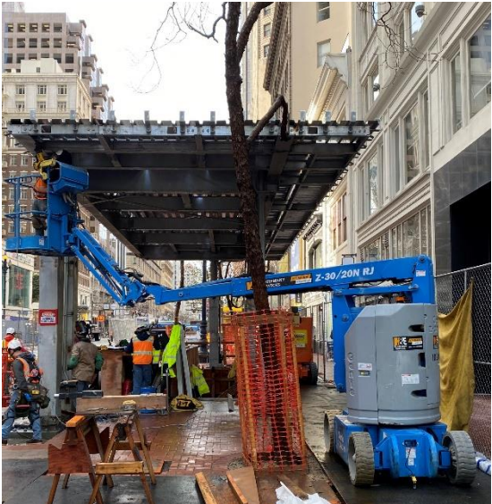
Metal Deck Installation
