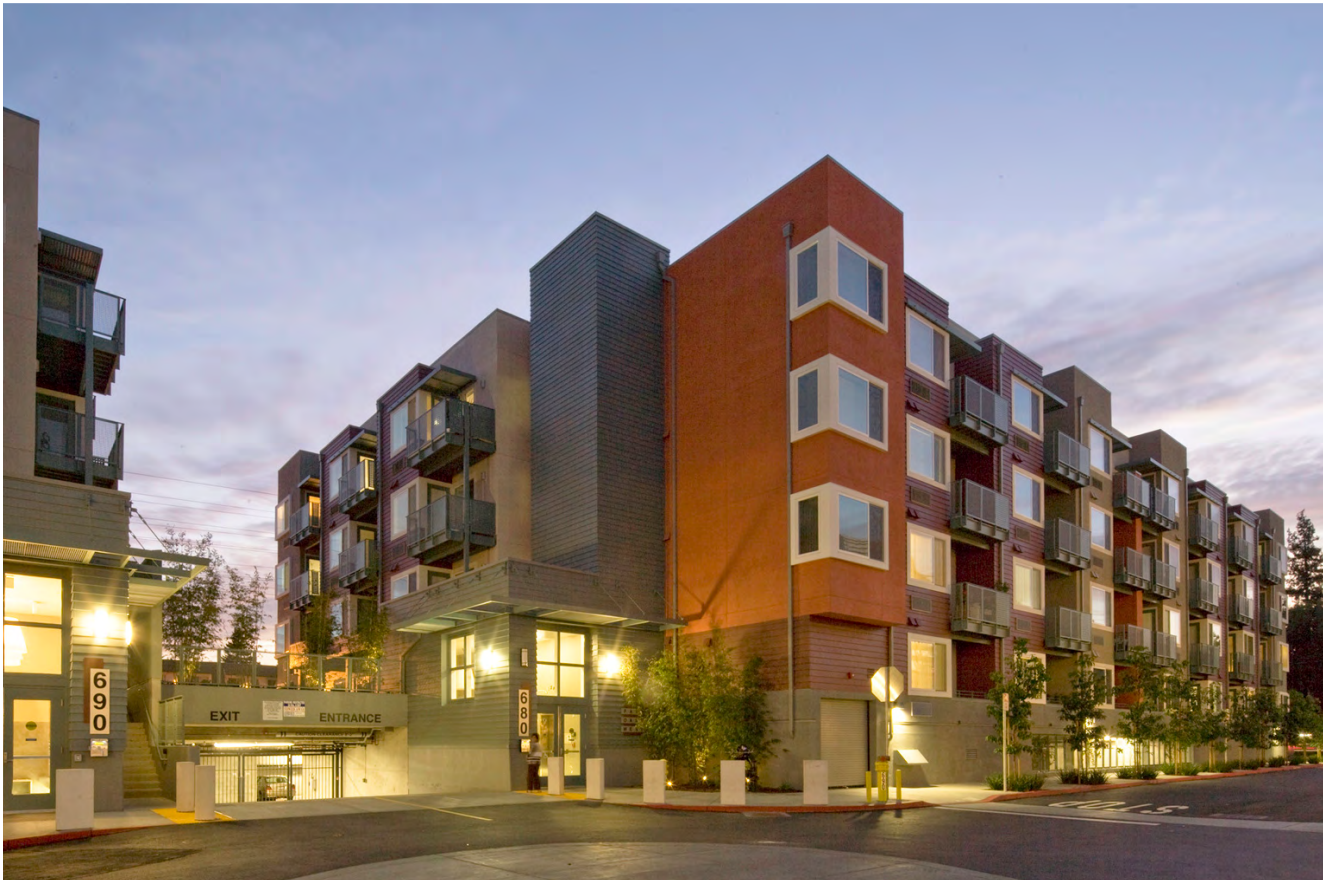
Fair Oaks Plaza apartments, Santa Clara County
