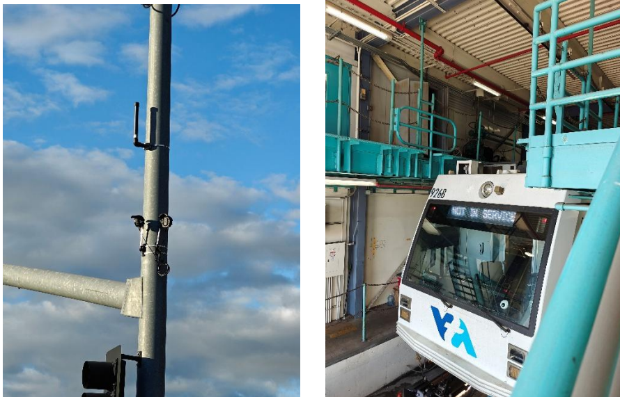
TSP equipment - intersection (left) and in-vehicle (right) installations. VTA Photos.
