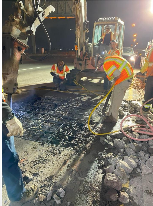
San Mateo-Hayward Bridge deck repair
