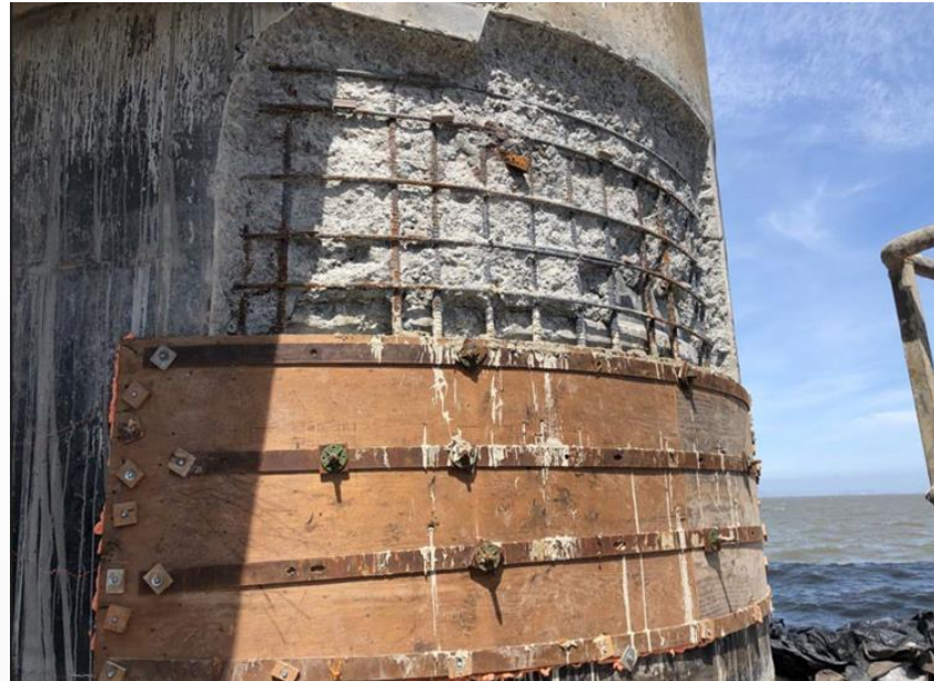
San Mateo-Hayward Bridge over water concrete repair
