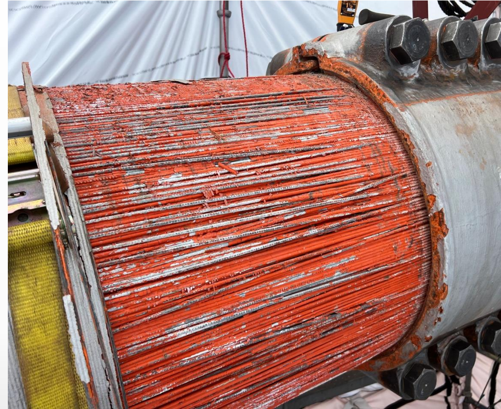
San Francisco-Oakland Bay Bridge West Span cable investigation
