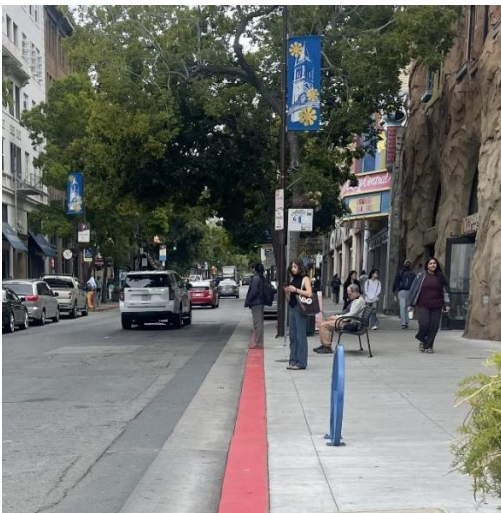
Telegraph Rapid Bus Stop Improvements. AC Transit Photo
