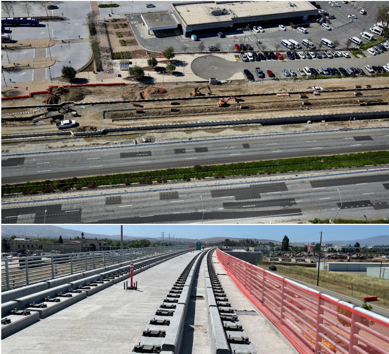
EBRC Construction progress – Top: Eastridge Station; Bottom: preparation for trackwork. VTA photos
