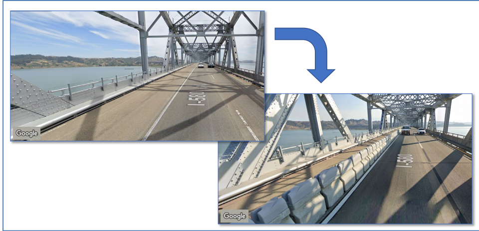
Figure 2-18: Upper Deck Modifications for the Bike/Pedestrian Path
