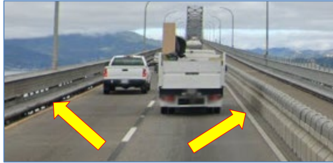
Figure 8-79: Relative Closeness Bridge Guardrail on the left and Path Barrier on the Right
