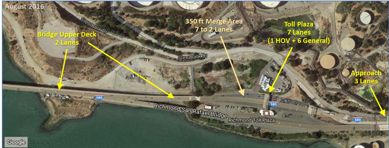
Figure 2-3: Initial Conditions – Westbound Bridge Approach in Richmond
