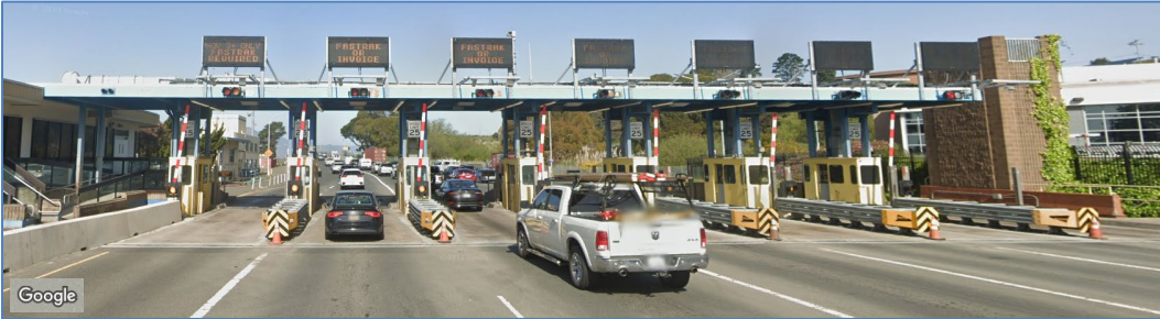
Figure 2-8: Approach to Richmond-Toll Plaza in April 2023
