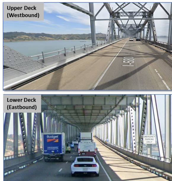
Figure 2-5: Initial Conditions – Bridge Upper and Lower Decks
