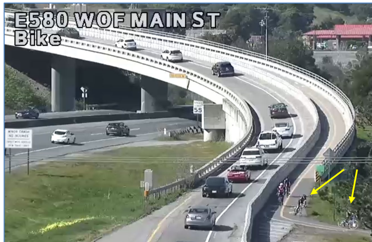
Figure 10-3: Riders Cutting Across Opposing Lanes at Bottom of Overcrossing
