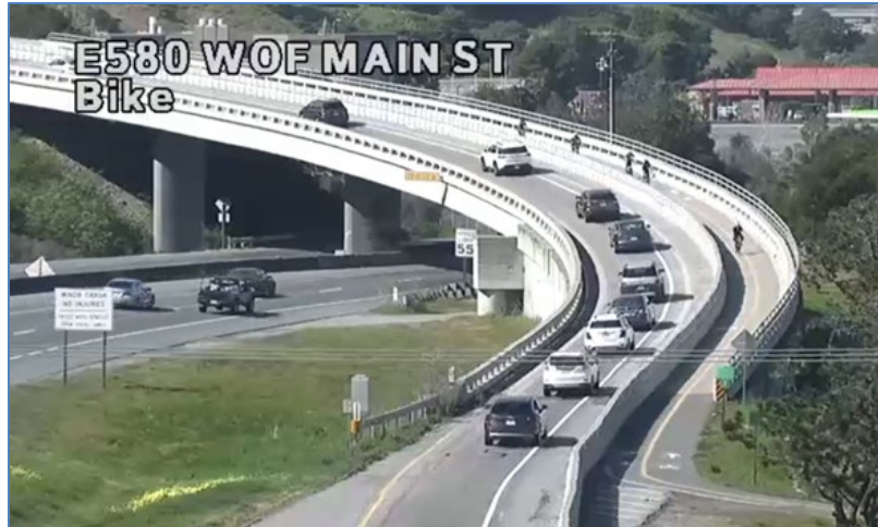
Figure 5-13: Pre-set View from Caltrans CCTV Camera
