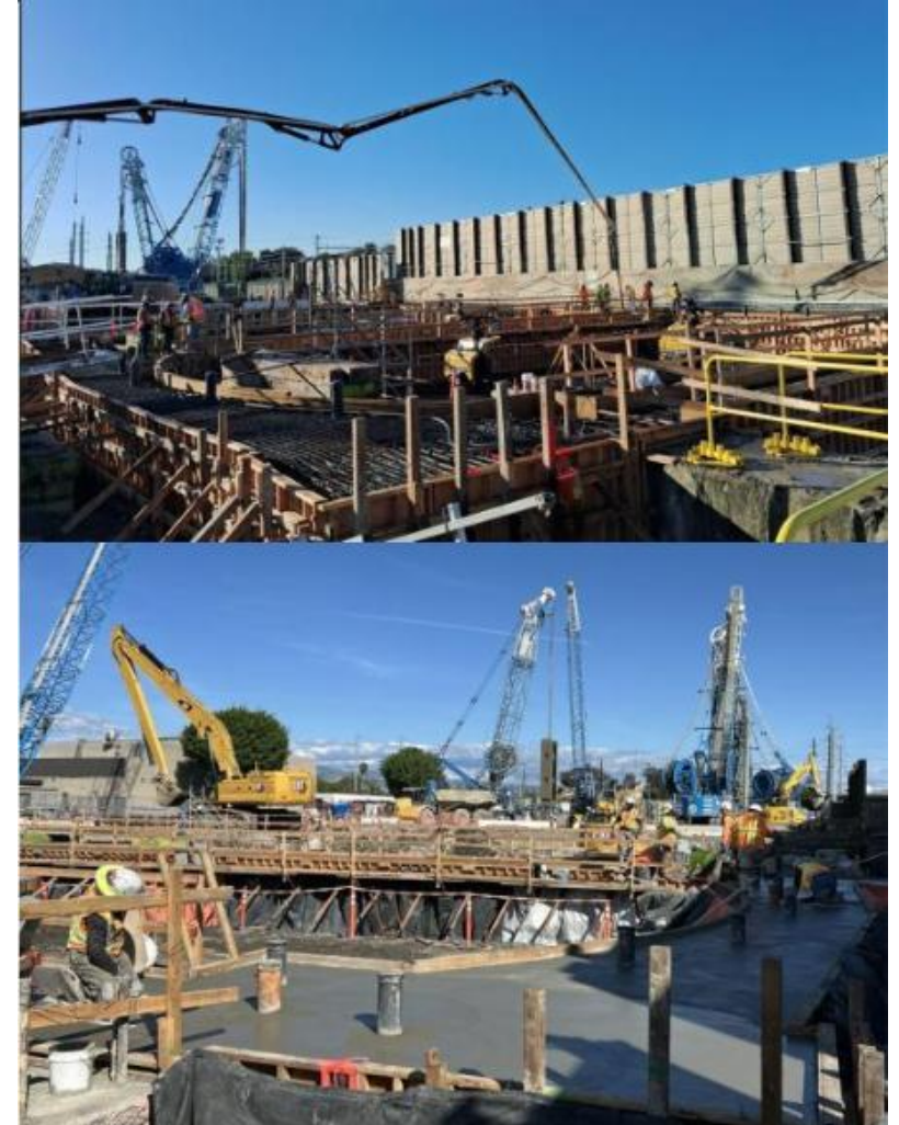
Photos: West Portal construction (VTA)
