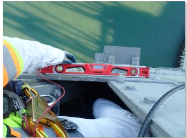
Figure 1-D: Physically measuring flatness
