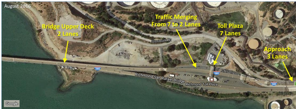
Figure 2-5: Initial Conditions – Westbound Bridge Approach in Richmond
