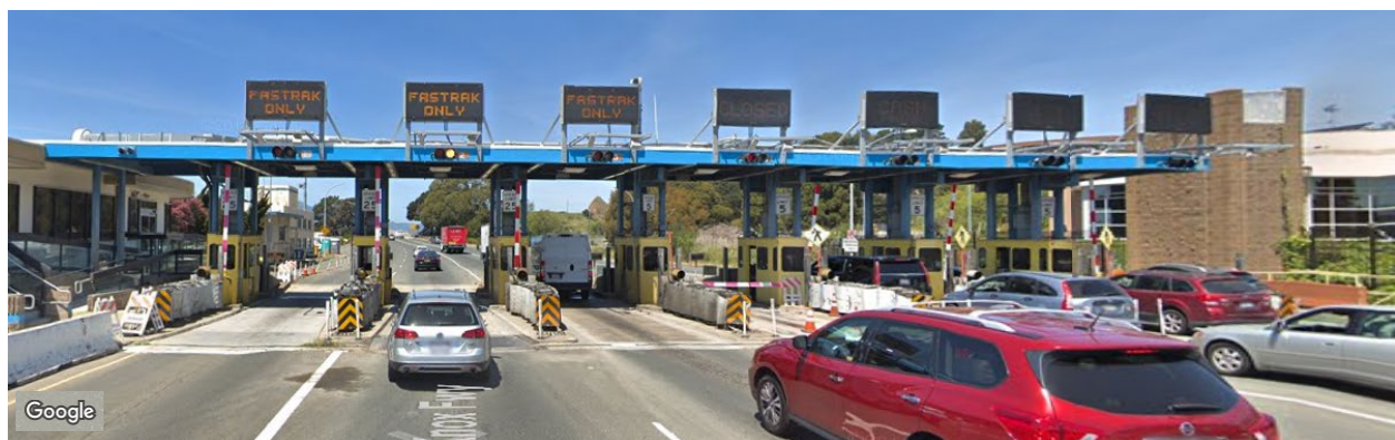
Figure 2-4: Approach to Richmond-Toll Plaza before March 2020
