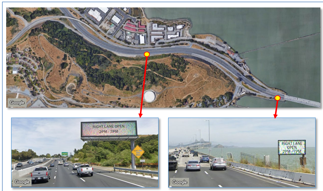
Figure 2-15: Dynamic Sign Indicating Shoulder Lane Open Status
