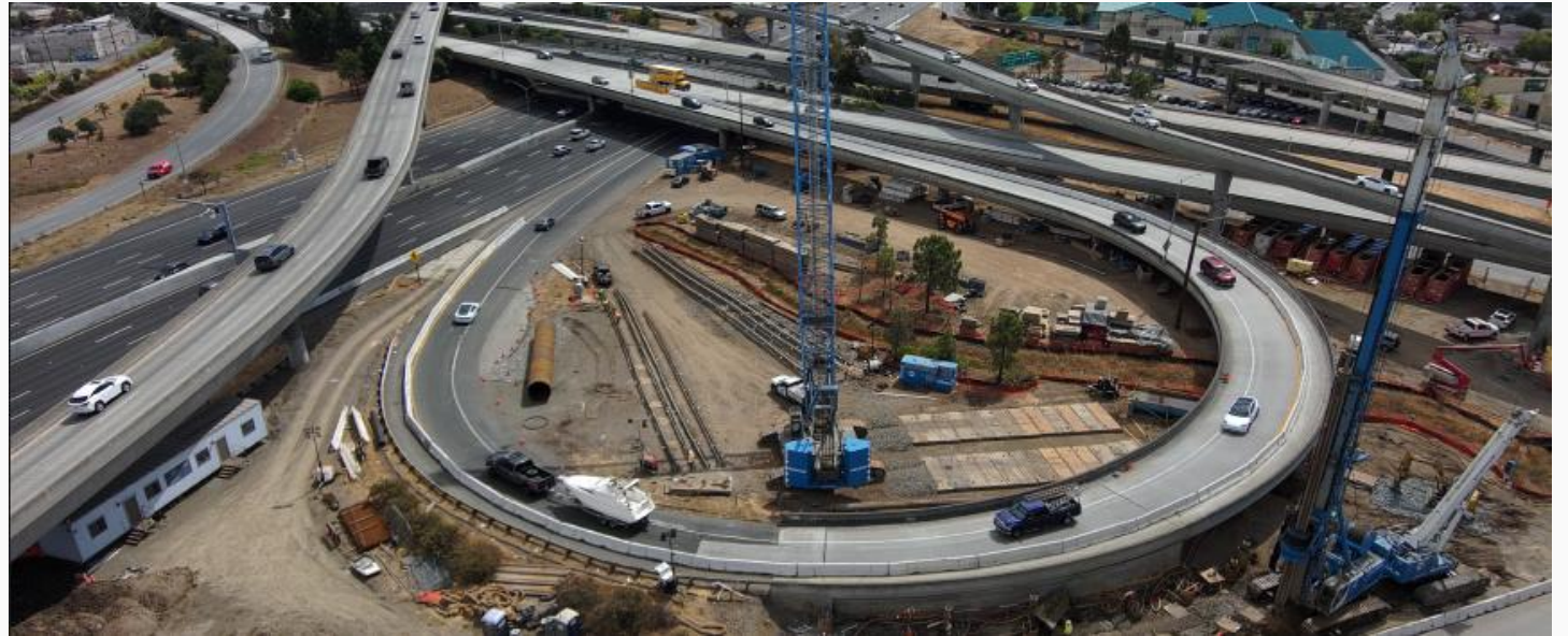
San Mateo US-101/SR 92 Area Improvements
