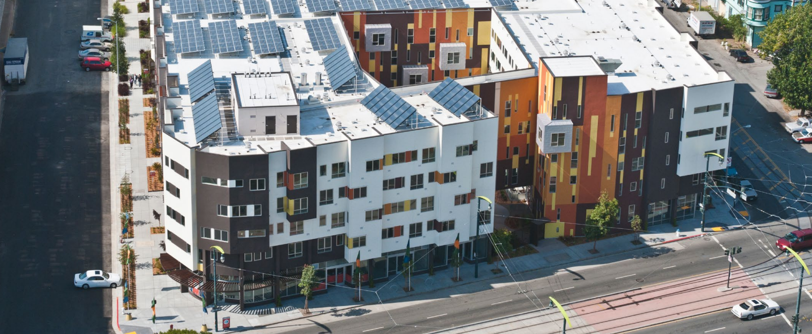
Armstrong Place Senior Housing and Armstrong Townhomes in San Francisco PHOTO BY STEVE PROEHL, COURTESY OF BRIDGE HOUSING
