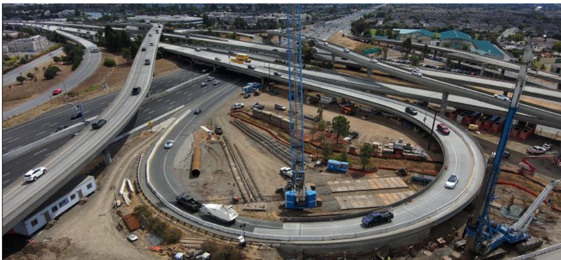
US 101/SR 92 Construction Progress SMCTA Photo
