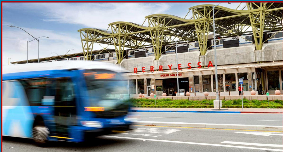
BART to Silicon Valley, Phase 1
