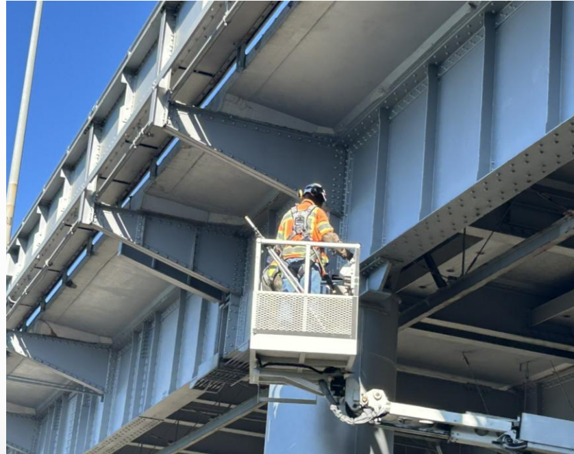
In-Depth Inspection of Important Steel Members
