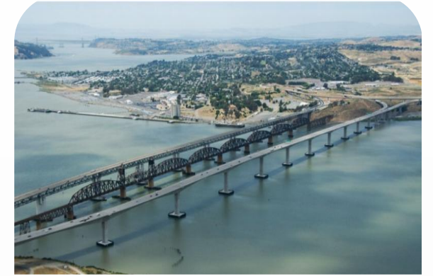
Benicia Martinez Bridge Southbound Opened: 1962 Northbound Opened: 2007
