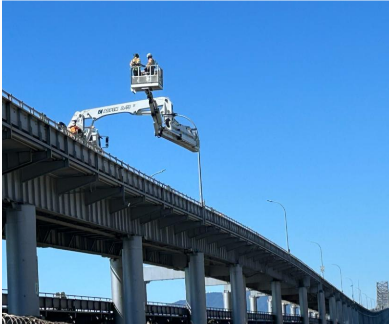
Under Bridge Inspection Truck (UBIT)
