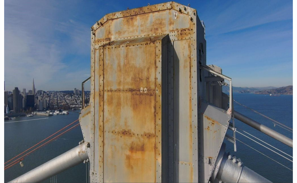
Steel Paint Projects for San Francisco-Oakland Bay Bridge West Span & Richmond-San Rafael
