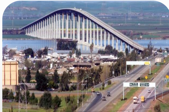
Antioch Bridge Opened: 1978
