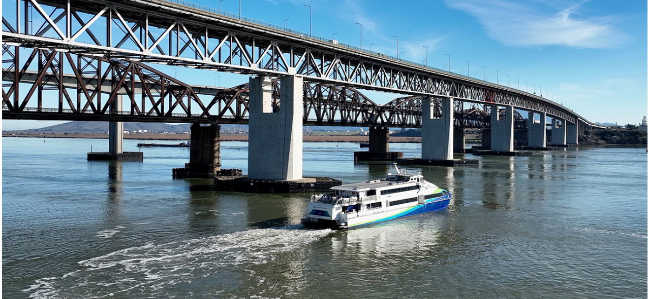
A WETA ferry carries state officials, BATA staff and others on an inspection tour of the Benicia-Martinez Bridge. Photo: Mark Jones, MTC
