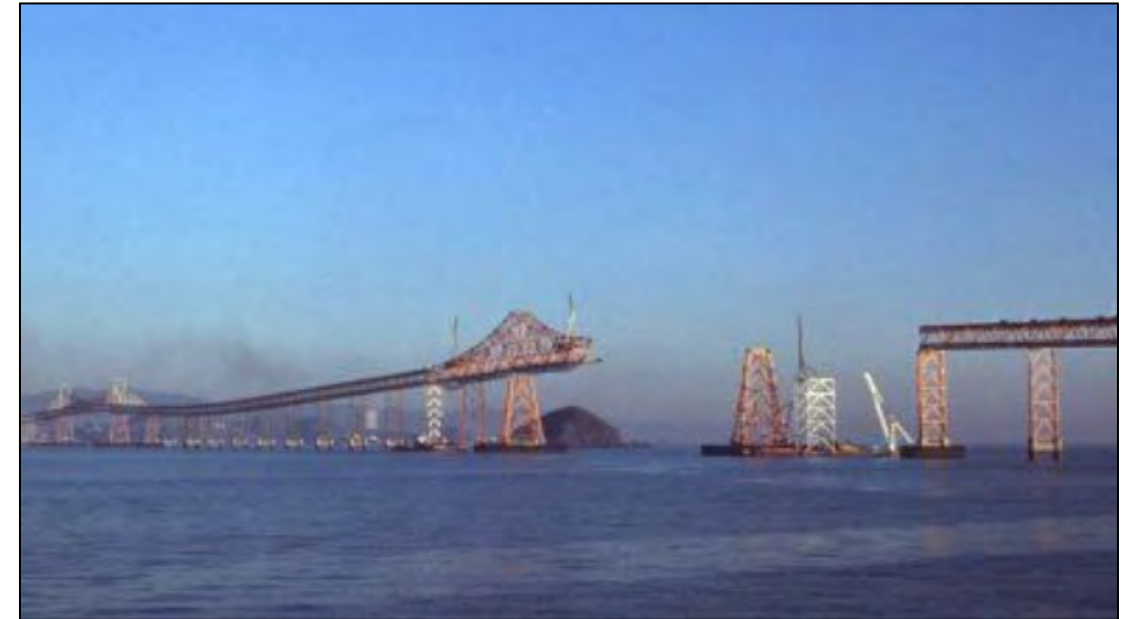
RSR Bridge: Opened in 1956
