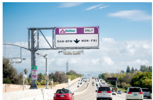
Overhead hours of operation sign and toll system equipment on the I-680 Express Lanes
