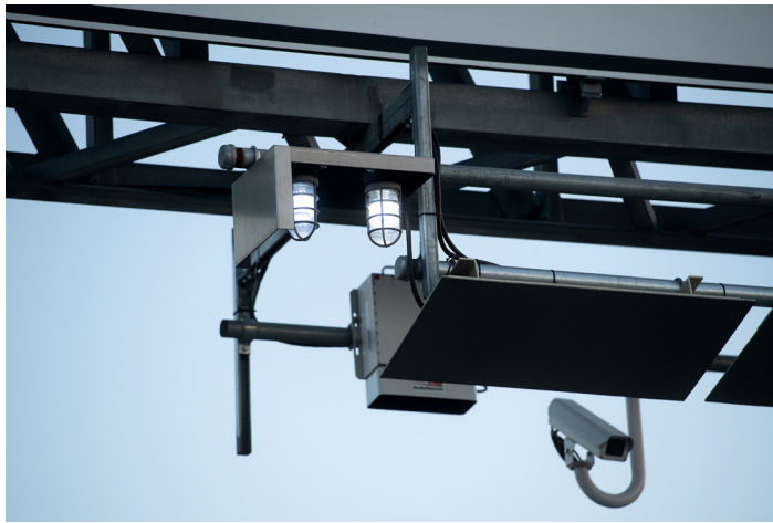
Close-up of toll system equipment under sign (enforcement beacons, reader antennae and laser trigger)
