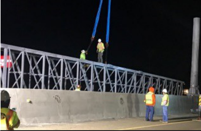
Offloading a new sign bridge on I-880 at West A St.
