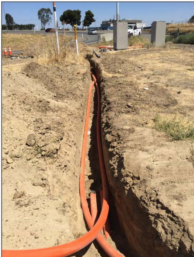
Backhaul trench to hub on I-680
