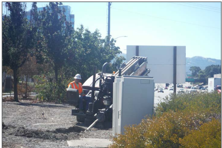
Crews boring conduit for the backhaul system. (See additional construction photographs on page 18)
