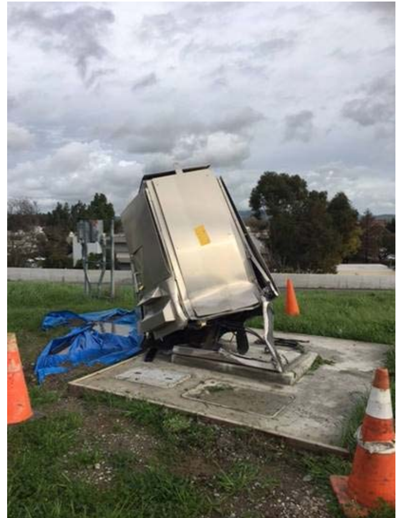
Damage to West Dublin cabinet from hit and run accident on 1/9/17
