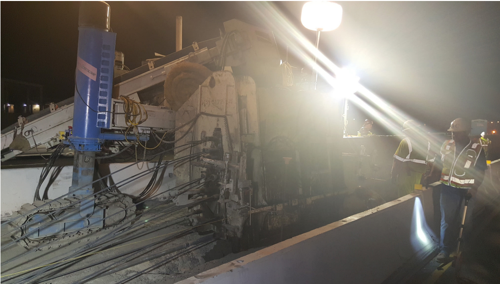
Slip form machine shapes concrete median barrier on I-880.
