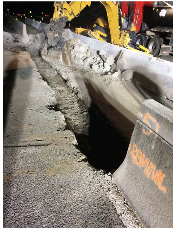
Median barrier demolition clean up.
