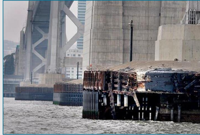
2007 Damaged SFOBB WS Fender
