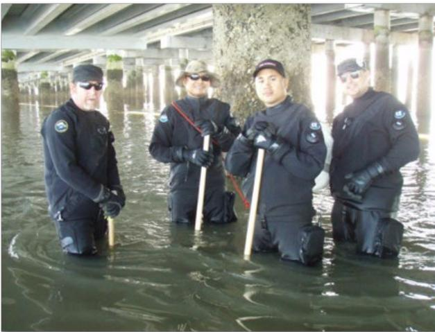
*Figure 1-C: Bridge underwater inspection*
