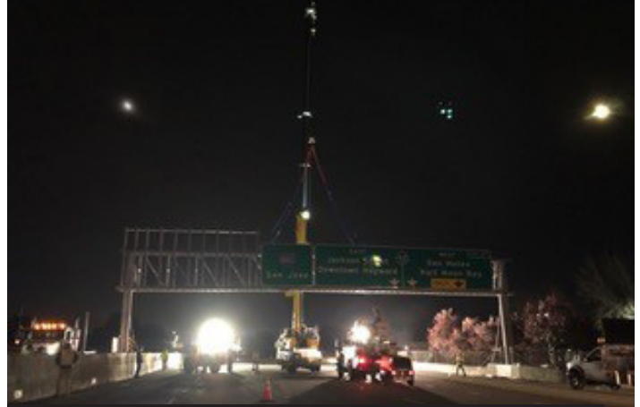
Erecting a new sign bridge on I-880 at Winton Ave.
