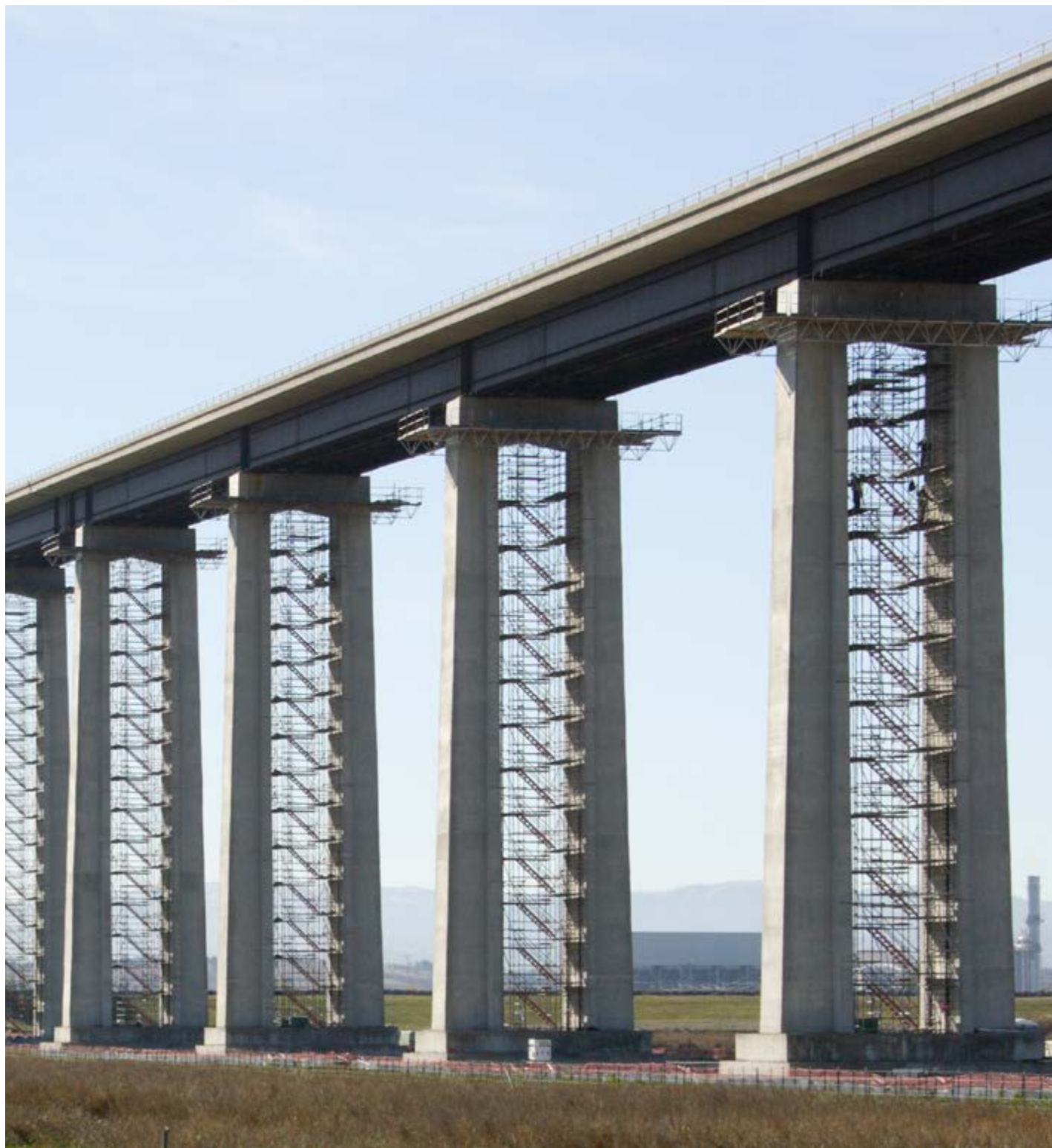
Seismic retrofit work on the Antioch Bridge, 2011
