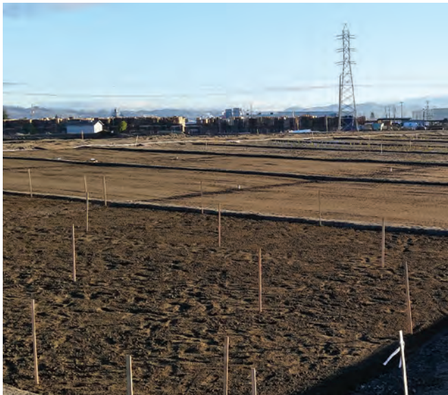
Photo, left: View of Horizontal Levee Demonstration Project at the completion of construction. The 400' by 150' demonstration is divided into twelve experimental cells with four different designs. Each design is built in triplicate to support research on the water quality, habitat, and hydraulic capacity of each Horizontal Levee cross section.
