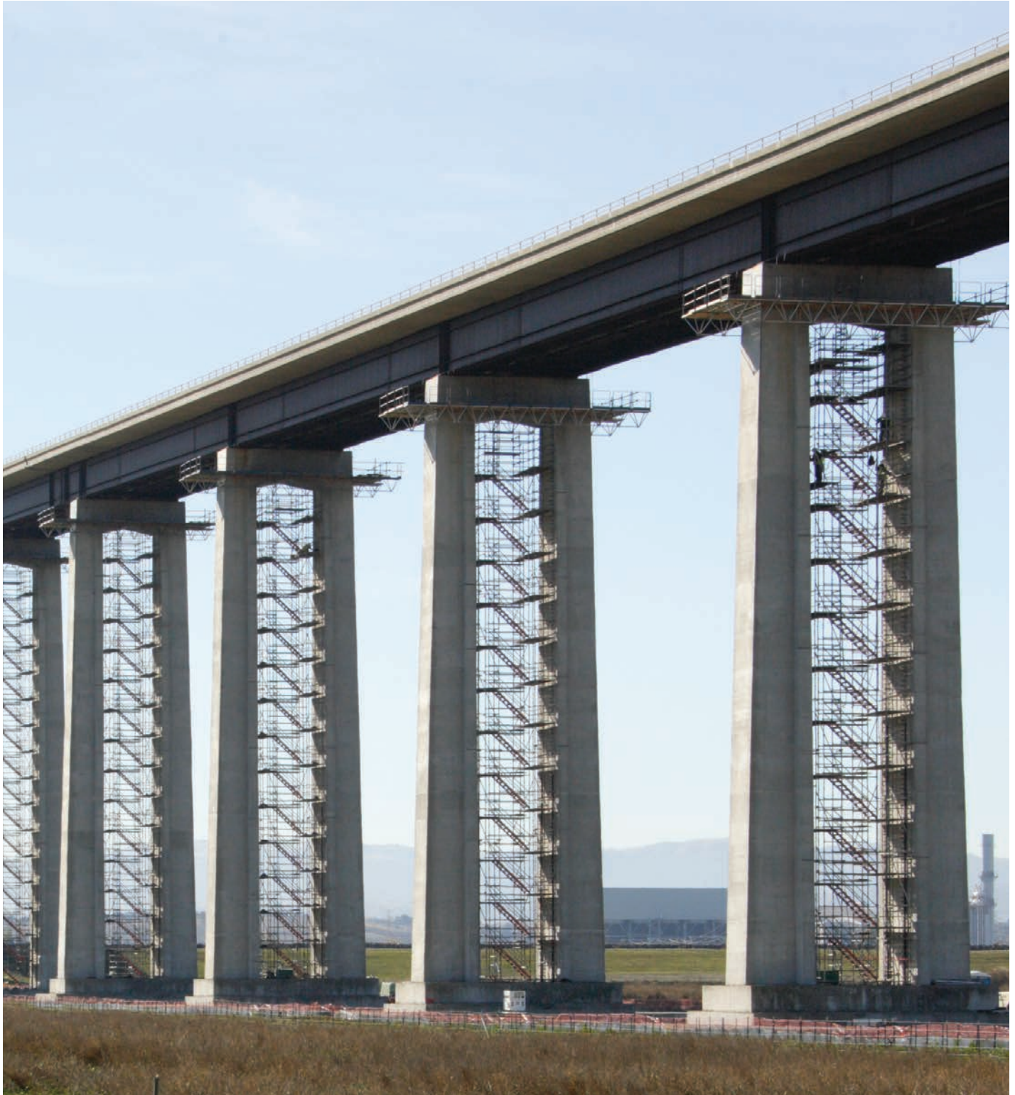
Seismic retrofit work on the Antioch Bridge, 2011
