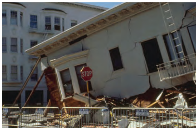
Liquefaction impacts in the Marina District from the 1986 Loma Prieta quake. Photo USGS
