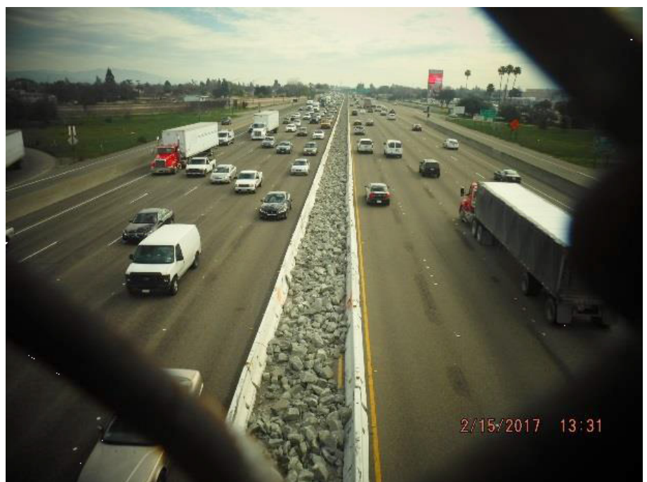
Demolished median barrier on I-880 near Winton Avenue in Hayward.
