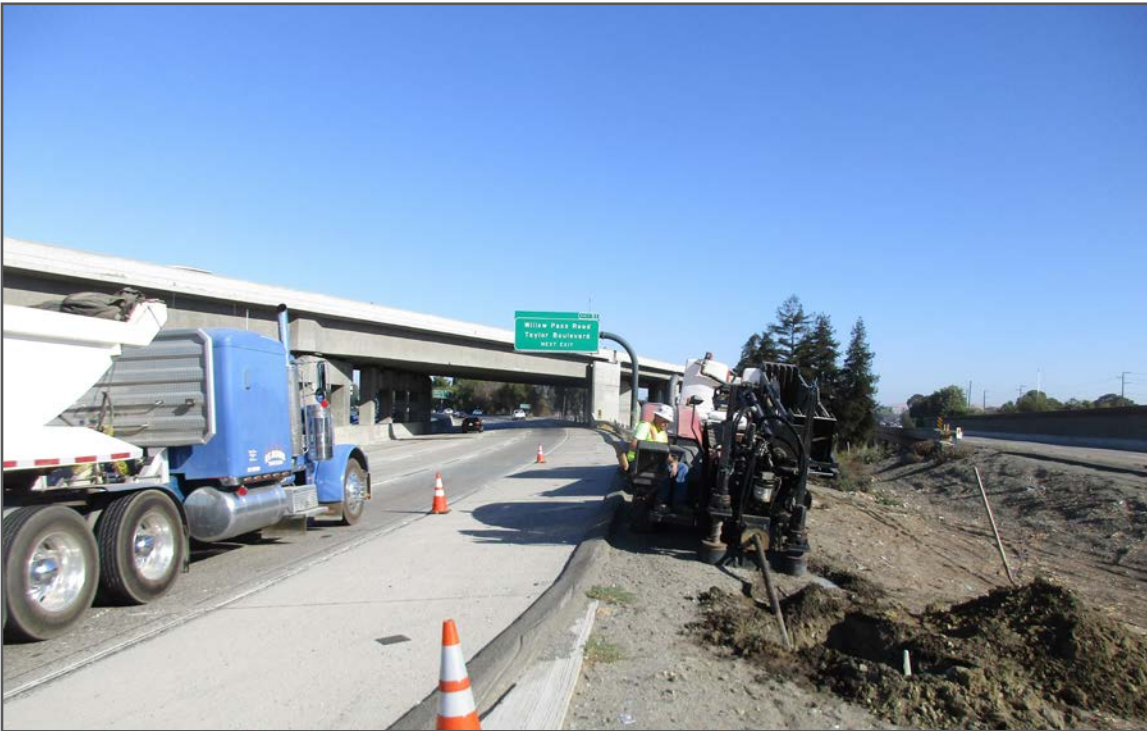
Backhaul conduit boring rig on I-680.
