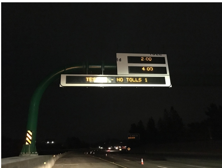
Construction crews testing an express lanes toll system sign on I-680.
