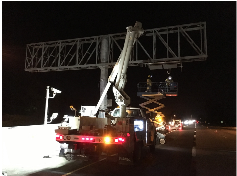
Crews install components of the toll system. (See additional construction photographs on page 19)
