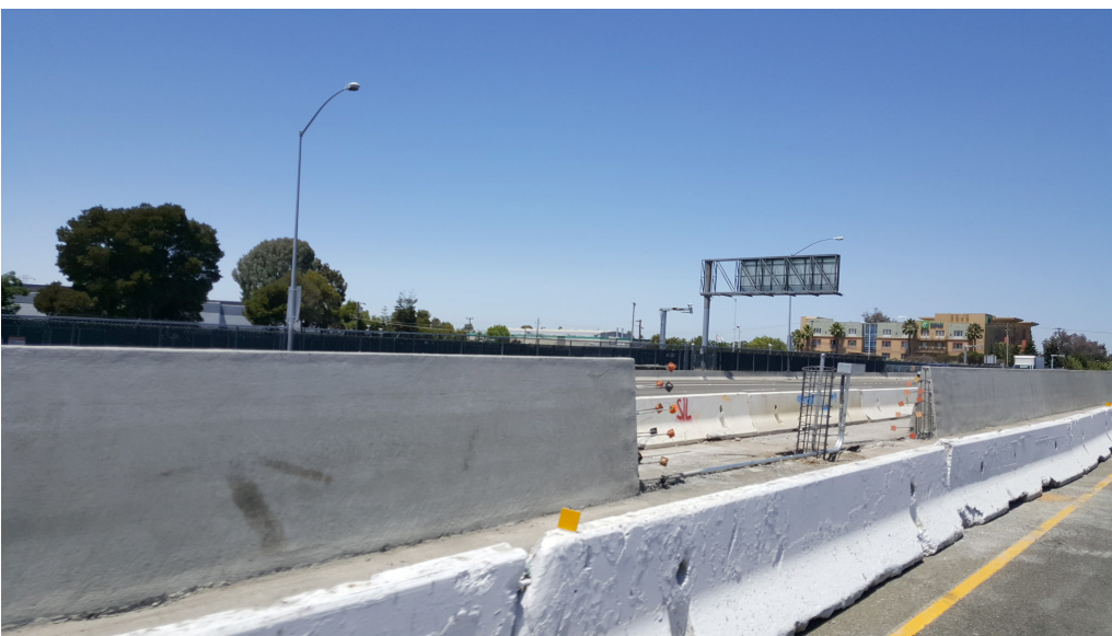
Gap in barrier along I-880 left by slip form/CIDH for lighting.
