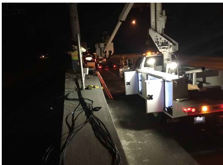
Construction crews install components of the toll system on I-680.
