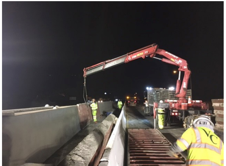
Installing forms for new barrier placement along I-880.
