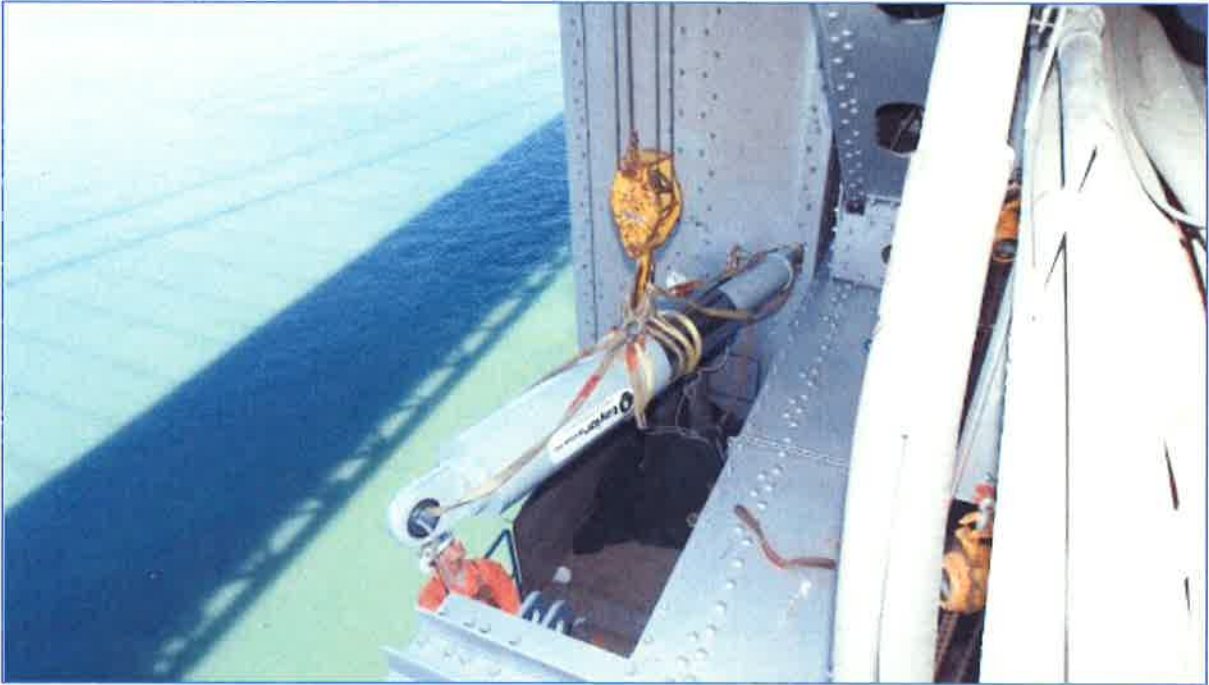
Photo of Installation of an Existing Damper
