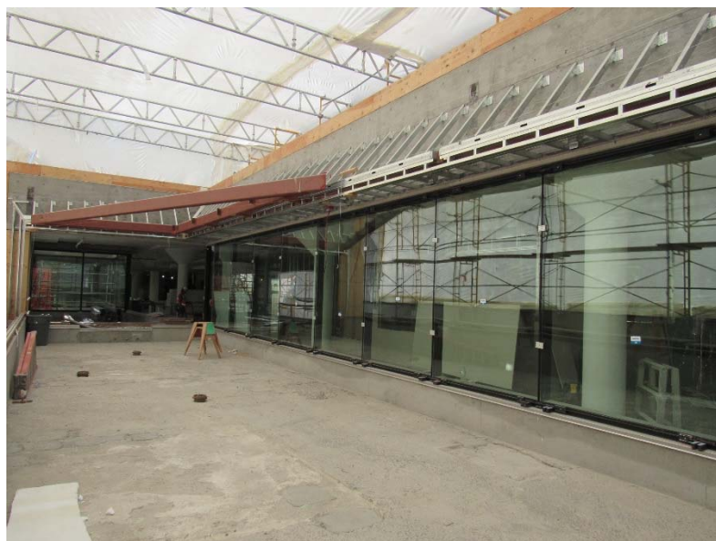
Figure 4: Level 8 terrace framing/glazing in progress
