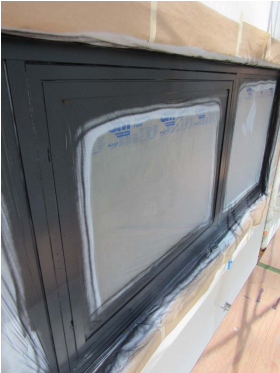
Figure 7: Exterior window painting in progress.
