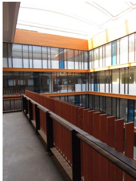
Figure 2: Atrium guardrail installation in progress.
