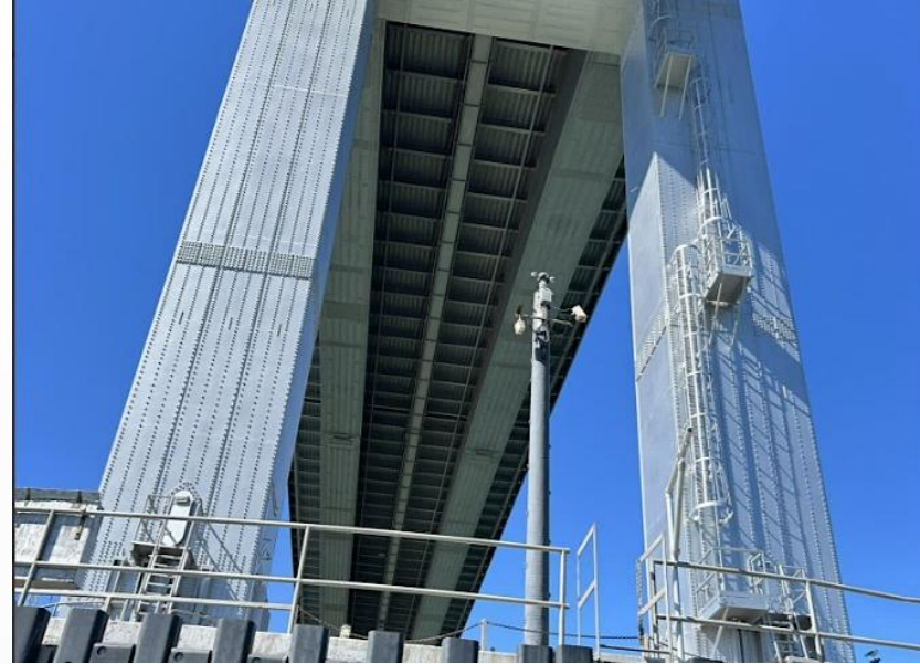
San Mateo-Hayward Bridge Tower Painting
