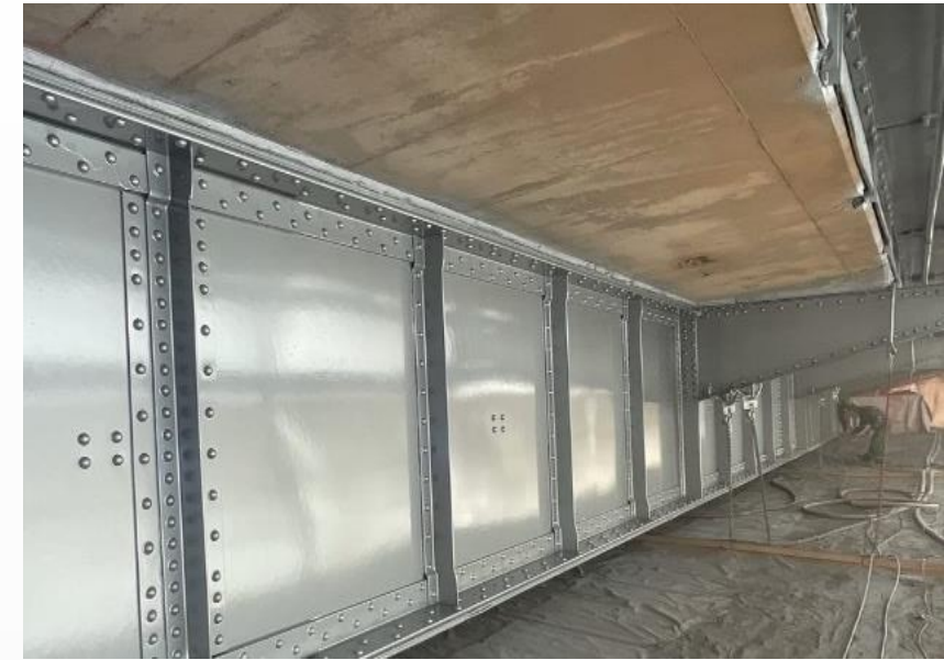
Richmond-San Rafael Structural Steel Painting
