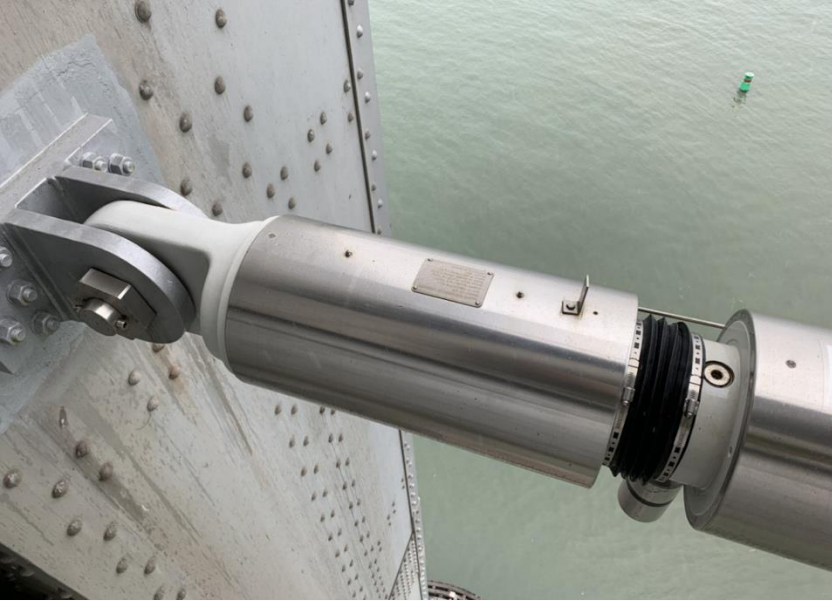
San Francisco-Oakland Bay Bridge Replace Seismic Dampers
