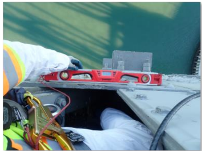
Figure 1-D: Physically measuring flatness
