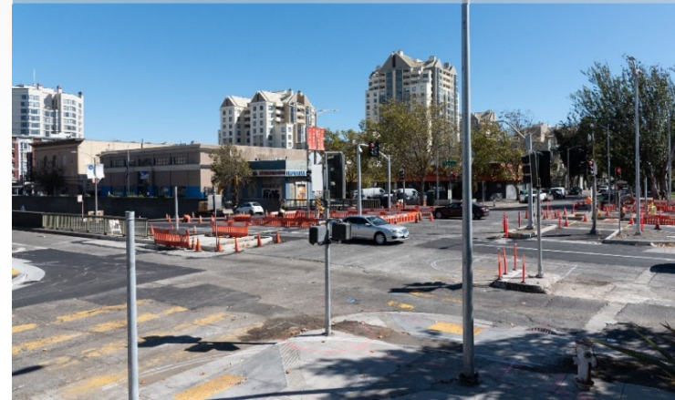
Geary Construction at Steiner
