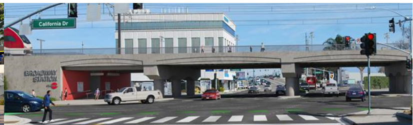
Grade Separation & Crossing Safety Upgrades
