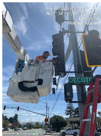
Dumbarton transit signal and TSP installation
