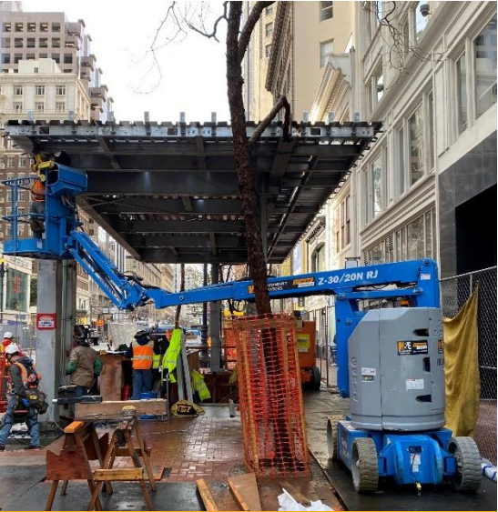
Metal Deck Installation
