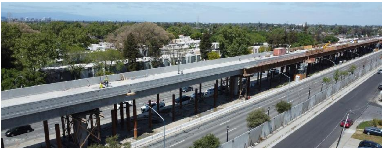
Aerial view of the Eastridge connector superstructure under construction. VTA images
