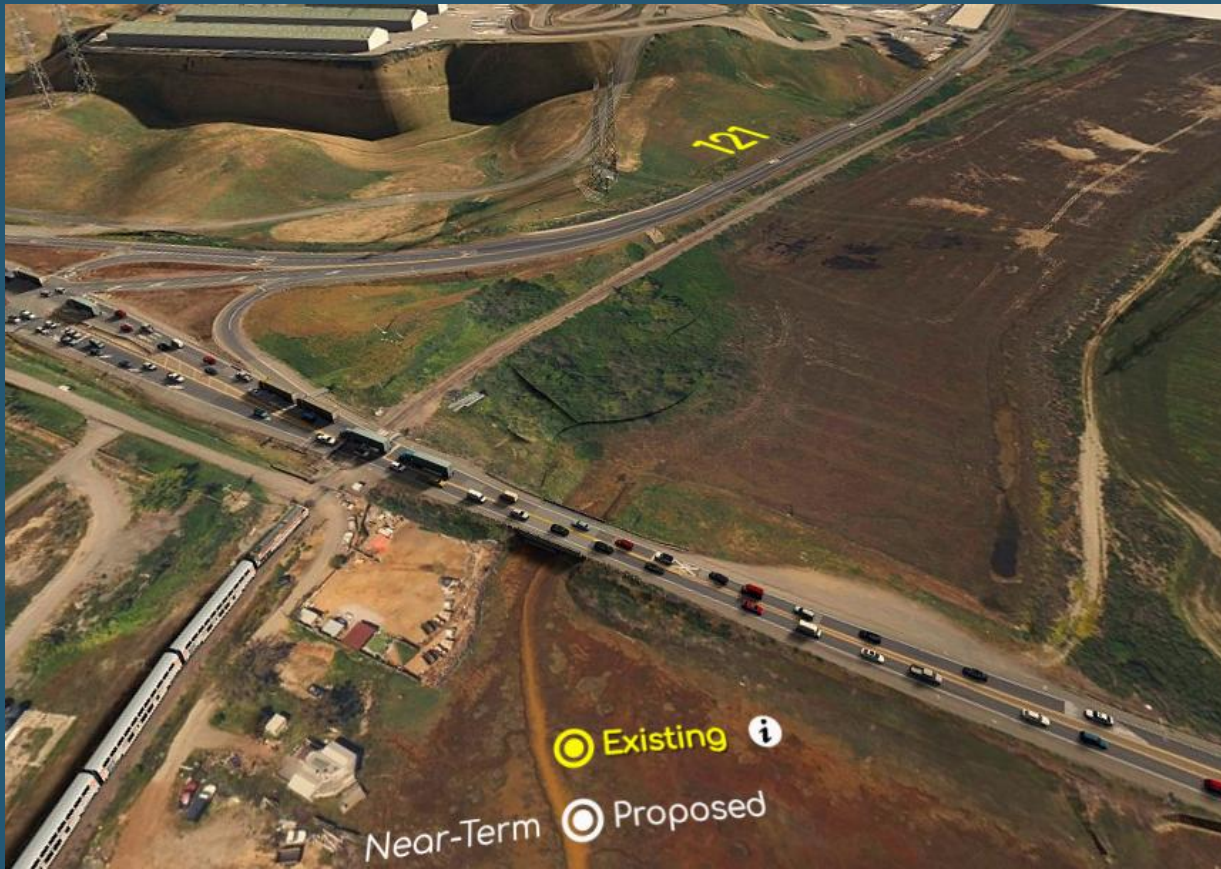
Existing Tolay Bridge
