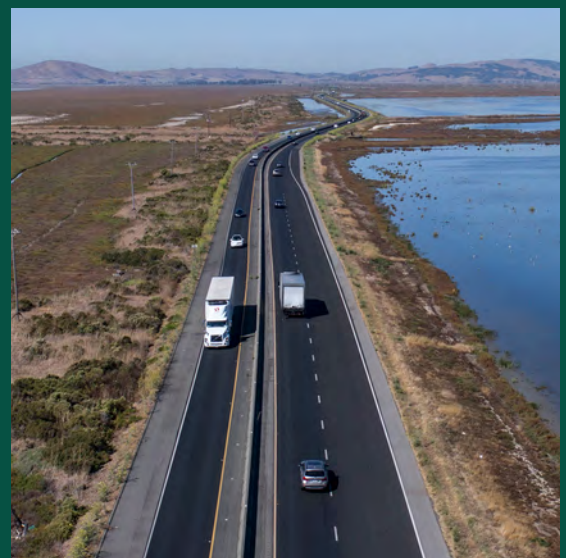
State Route 37 is a linchpin for the Bay Area economy. Photo: Karl Nielsen.
