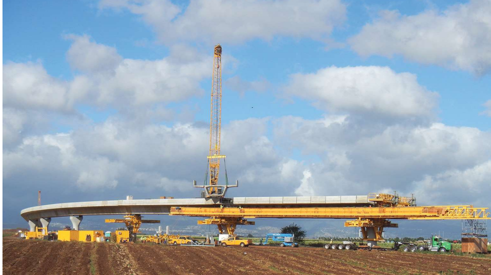
First 110 spans completed in the East Kapolei section of the project were built using the span-by-span erection method with a deck-mounted crane.
