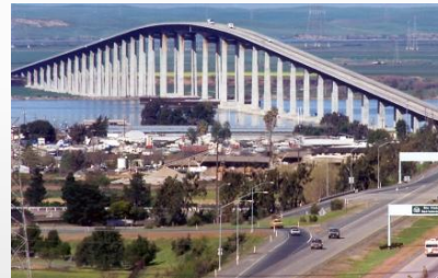
Antioch Bridge Opened: 1978
