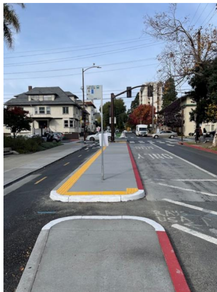
Photo: Completed bus boarding island on Dana St., part of Telegraph Rapid Bus Upgrade project, AC Transit Photo
