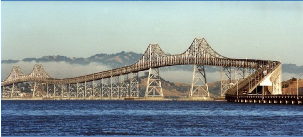
Figure 2-2: Richmond-San Rafael Bridge
