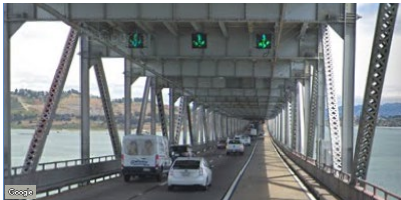
Figure 2-13: Electronic Lane Control Signs on Lower Deck
