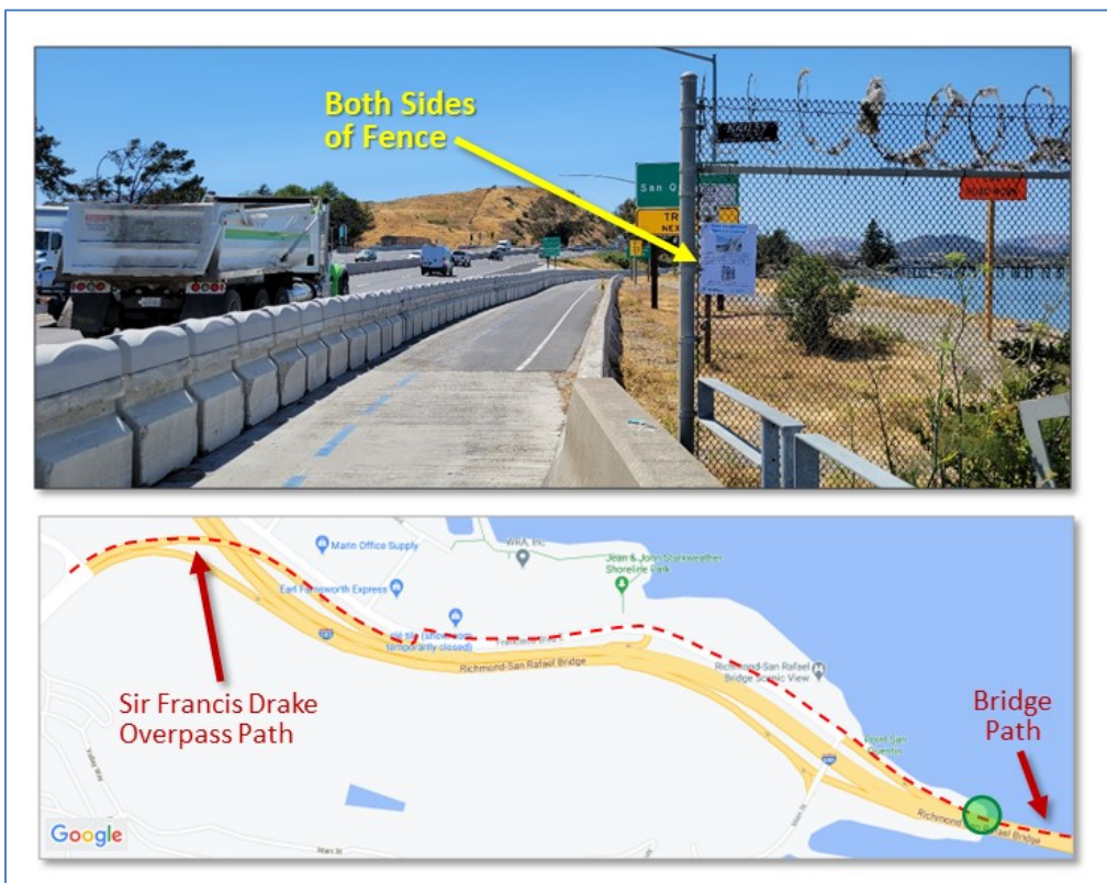
Figure 5-21: User Survey Signs Along Path – Marin County Side
