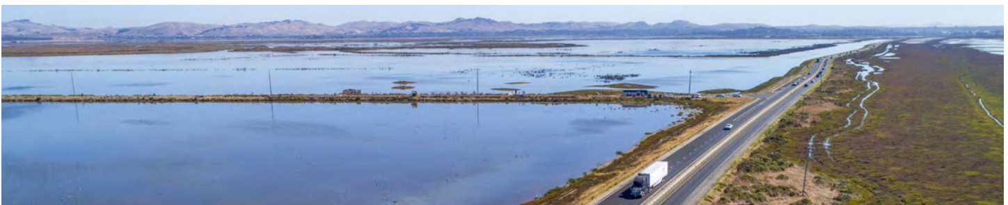
Preliminary cost estimates for just one regional adaptation priority — elevating the 21-mile State Route 37 corridor — are at least of $10 billion. Photo: Karl Nielsen.
