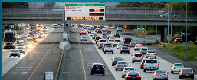
Bay Area Forward optimizes existing infrastructure to deliver low-cost, high-impact congestion relief through operational efficiencies.
