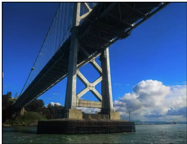
The Bay Bridge's western span will need several upgrades and repairs, including the fenders at the base of the piers.
